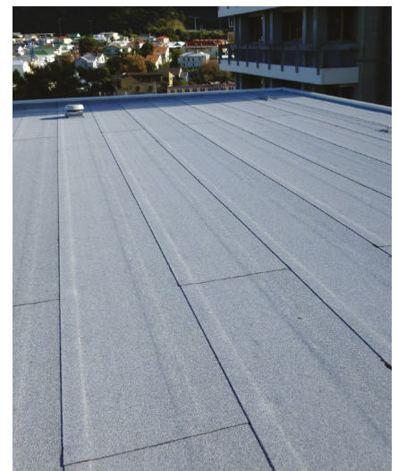
Multi-layer membrane roofing.
