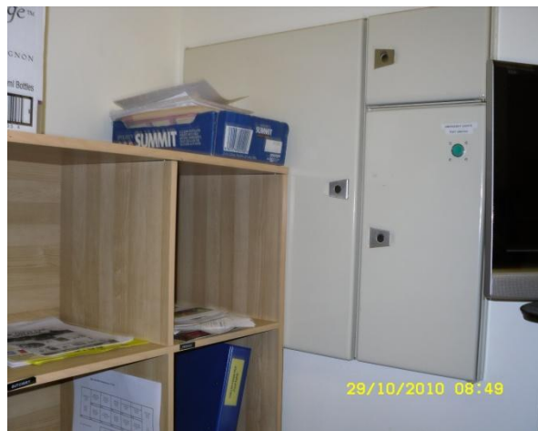
Figure 25. Board blocked by shelving installed after building completion
