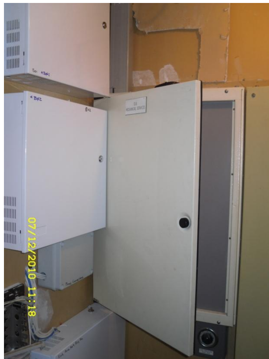
Figure 26. Board blocked by security panels
