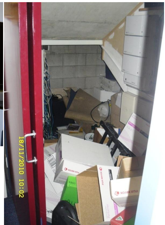
Figure 27. Board blocked by a jumbled storage area, both a fire and access hazard
