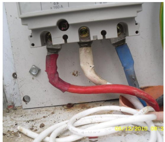
Figure 16. Melted insulation and exposed terminals. The building was newly wired
