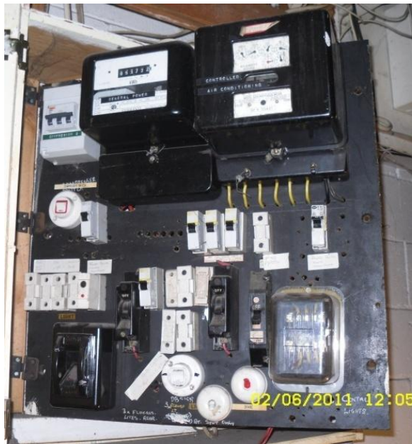
Figure 28. Typical reconfigured, older distribution board
