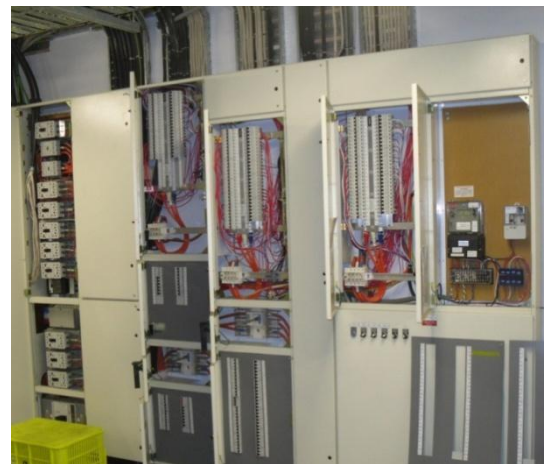
Figure 37. Large multi-panel distribution board showing circuits for end-use monitoring.
