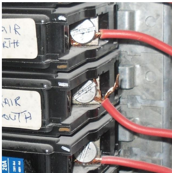
Figure 16. Melted insulation and exposed terminals. The building was newly wired
