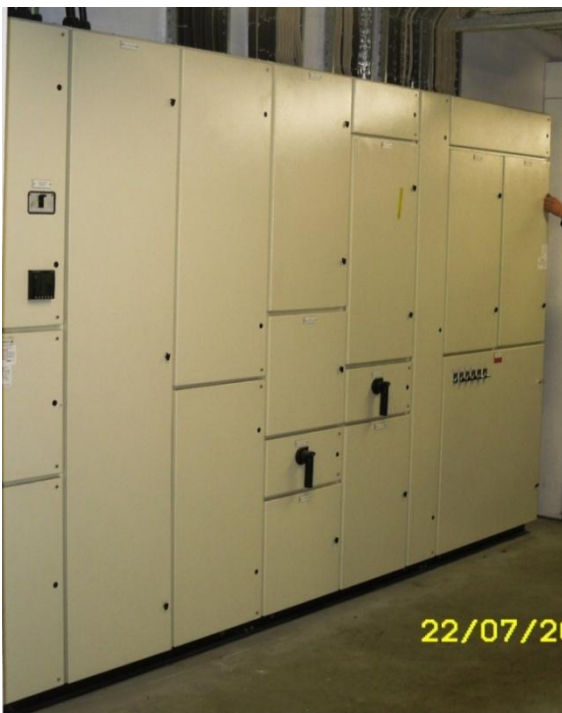
Figure 35. Large multi-panel distribution board.
