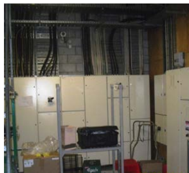
Figure E-19: Large Multi-Panel Distribution Board.
