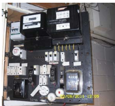
Figure E-16: Typical Reconfigured, Older Distribution Board.
