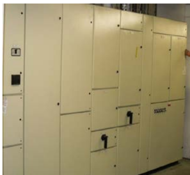
Figure E-18: Large Multi-Panel Distribution Board.
