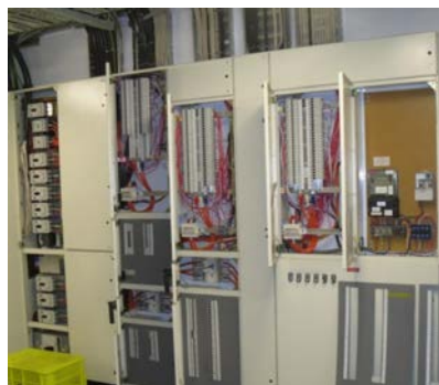
Figure E-20: Large Multi-Panel Distribution Board showing Circuits for End-Use Monitoring.
